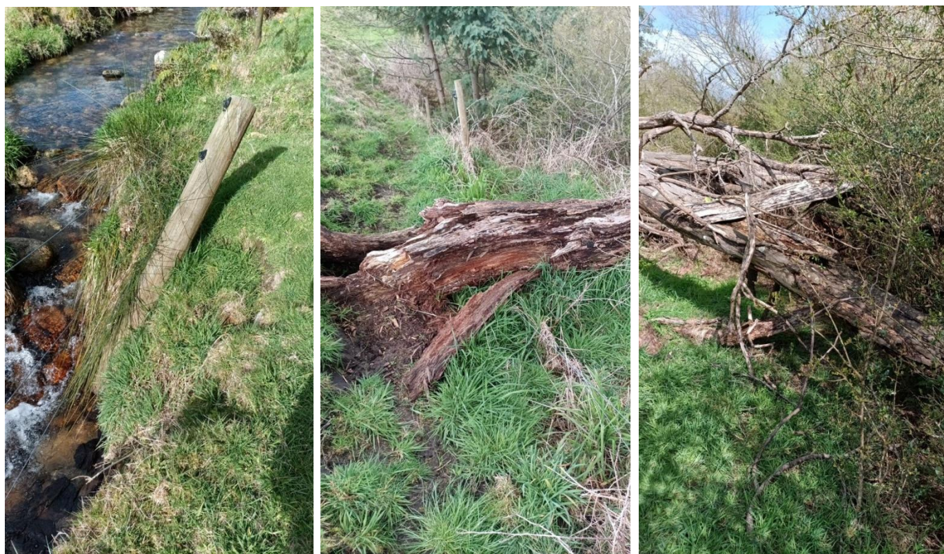
Figure 1 Photo 13,14,&15: Damaged fence lines
